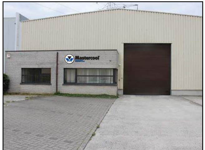
European Sales Office and Warehouse
